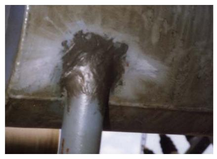
In a transformer station plant oil leakages at welding seams of a conservator were repaired with the Direct-MM-Bonding method by using MM-metal oL-steelceramic, Hardener red and Hardener yellow.
