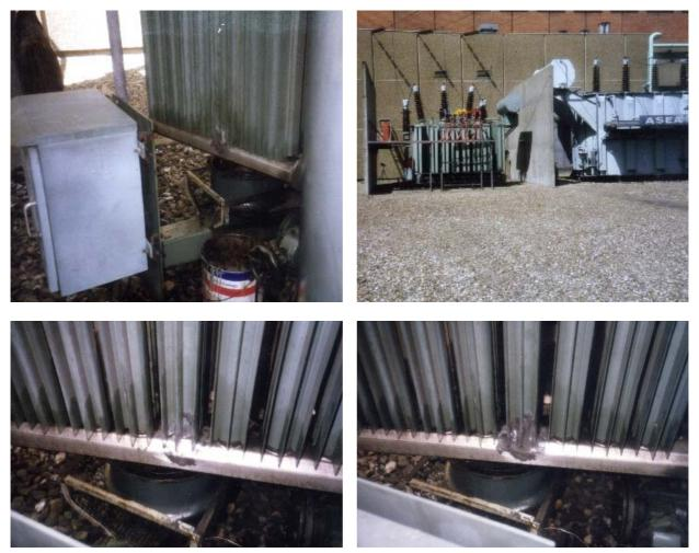
Sealing of a large transformer in a power station. The leakage was sealed with MM-metal oLsteelceramic and Hardener red using the Direct-MM-Bonding method. Then a layer of MMmetal oL-steelceramic and Hardener yellow was applied to the first layer.
