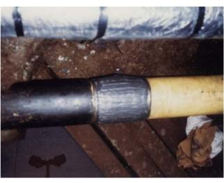
A leakage in a 154 KV P.O.F. insulation pipe was sealed using MM-metal oL-steelceramic and Hardener red working with the Direct-MM-Bonding method. In addition corrosion damages of the piping were removed by applying MM-metal SS-steel, liquid and Hardener yellow, liquid. Oil pressure 200 psi, diameter of the piping 300 mm, oil quality polybdenum.
